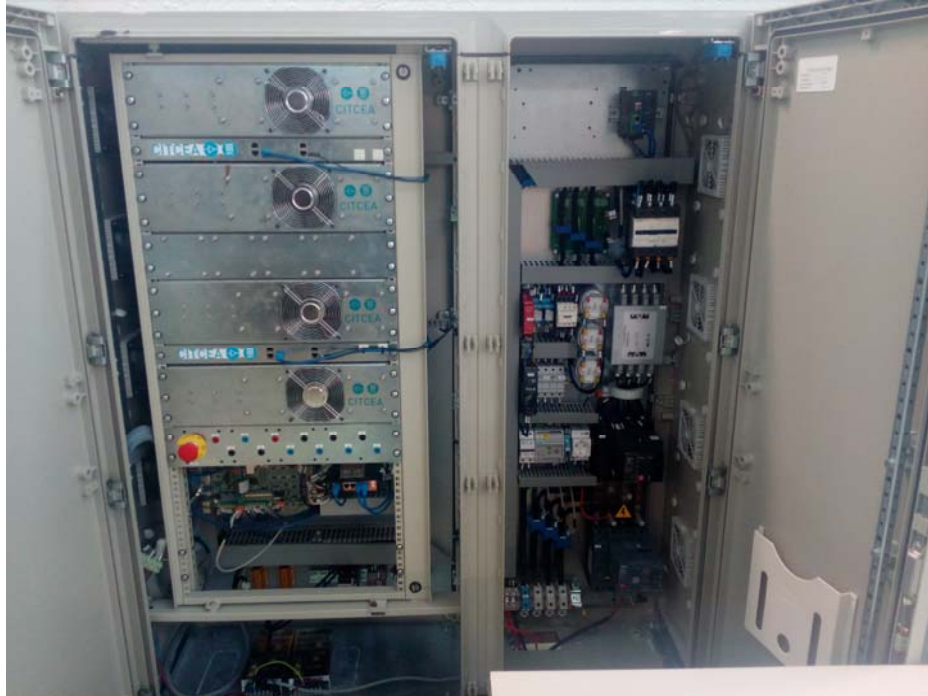
Figure 15. Bidirectional voltage source converter utilized for testing the lithium-ion battery pack.
